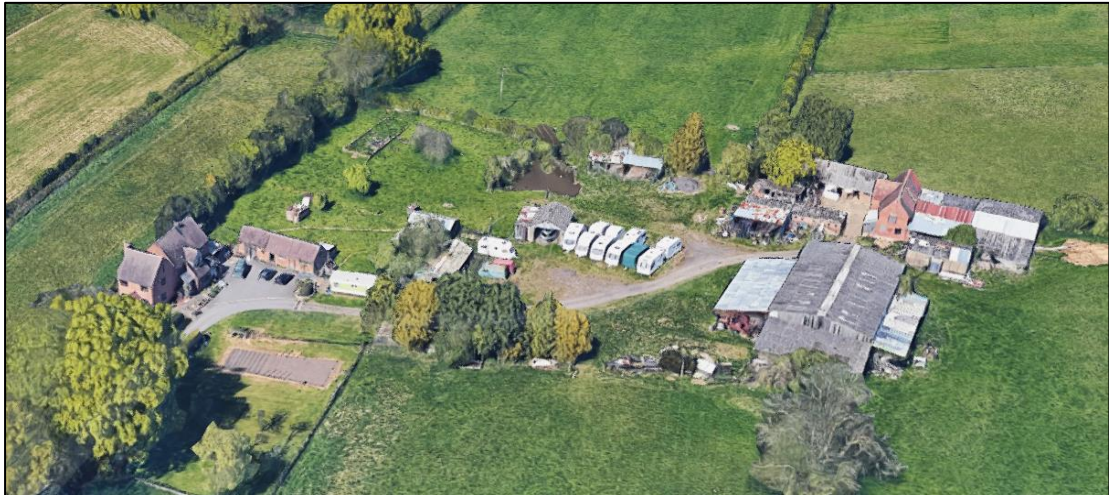
Figure 15: Grade II listed Hillside Farm
