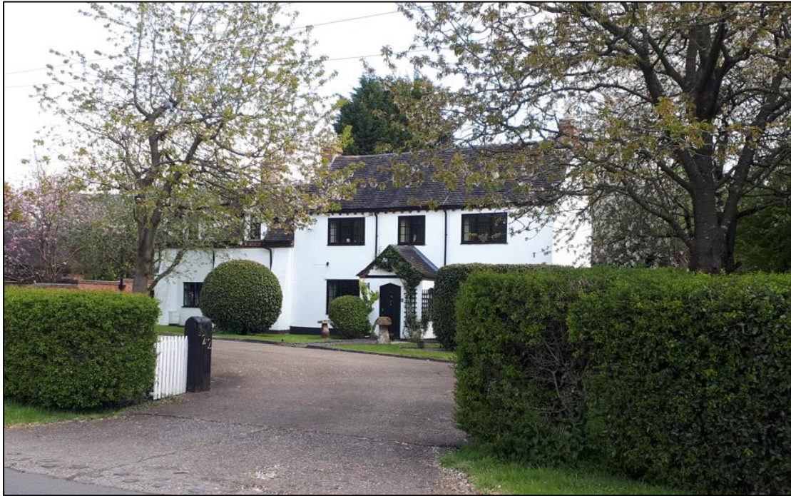
Figure 17: Grade II listed 122 Wall Hill Road
