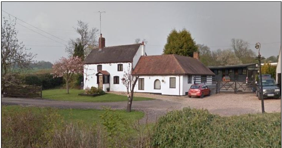
Figure 18: Grade II listed 128 Wall Hill Road
