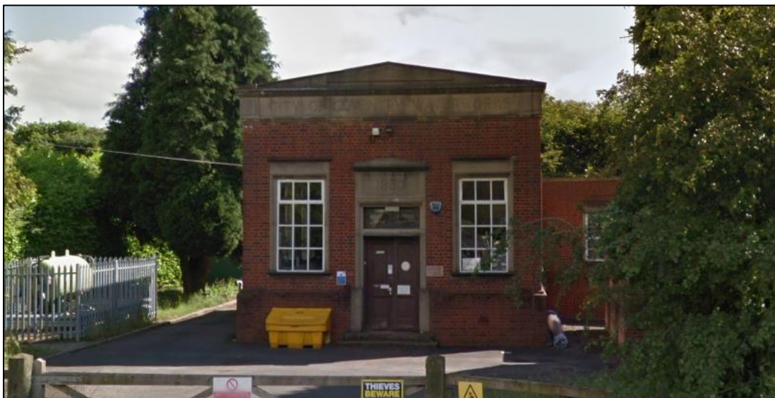
Figure 14: Locally Listed Pumping Station
