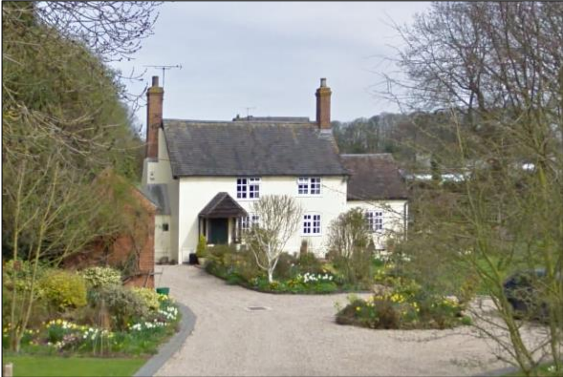
Figure 16: Grade II listed 112 Wall Hill Road
